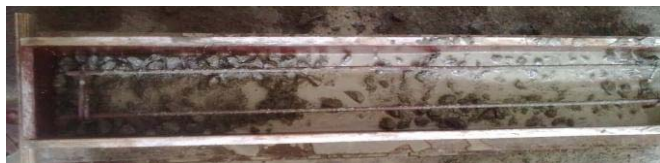
Fig. 7 Casting of beams - Shear
