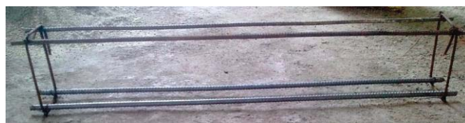
Fig. 5 Reinforcement cage - beams in shear
