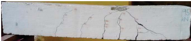
Fig. 16 Crack pattern of MKB-S
