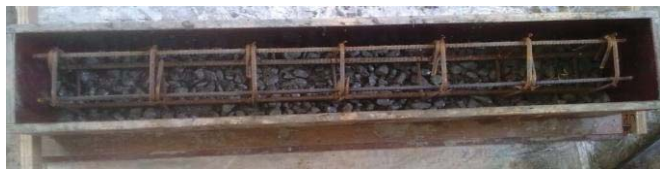
Fig. 6 Casting of beams – Flexure
