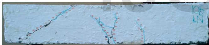
Fig. 18 Crack pattern of MKHSFB-S
